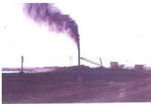
FIG. (22-D) THE FIRE HAS BEEN SUCCESSFULLY EXTINGUISHED AND THE WELL HEAD IS PREPARED FOR CAPPING.
